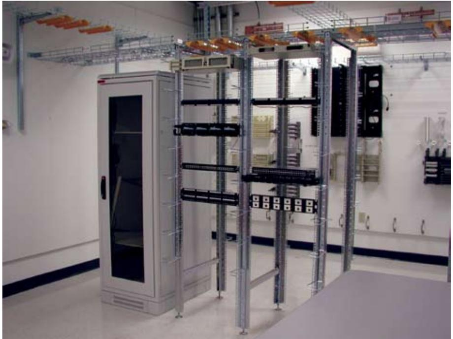
**In the BICSI Tampa Training Center, the Defem concept was built as one mechanical structure to support the cable channeling and to serve as support for the open integrated racks. Complete flexibility to use either cabinets or open racks under the Multi-Level Cable Channel structure.**
